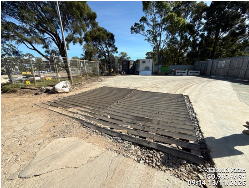
Photo 19 Rumble Grid Was Installed
