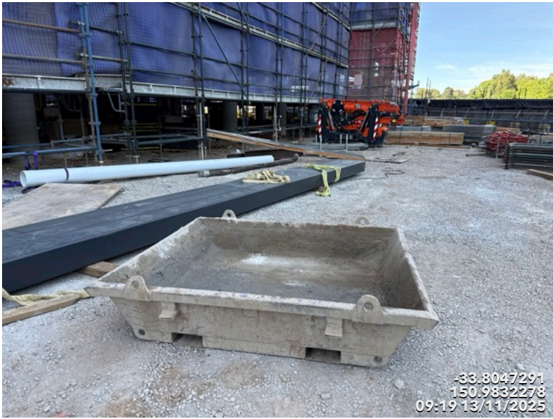
Photo 27 Concrete Washout Tray
