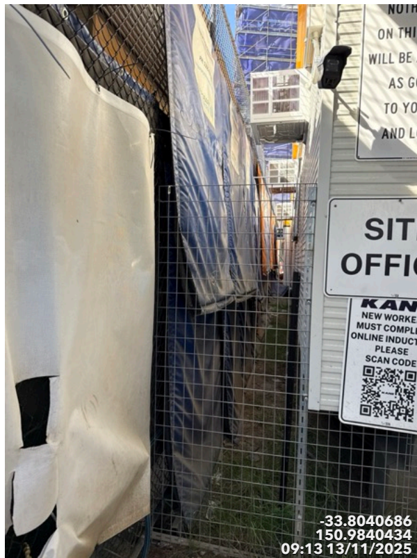
Photo 18 Acoustic Pads were Used
