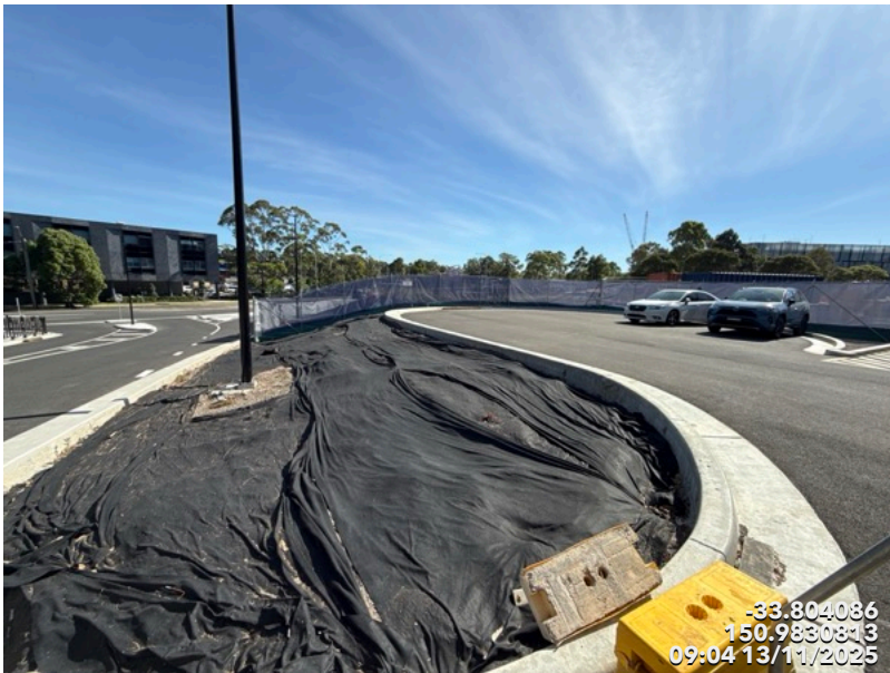
Photo 4 Ground covered with geofab.
