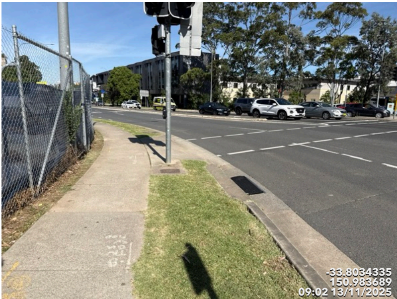
Photo 2 Pits covered with geofab.
