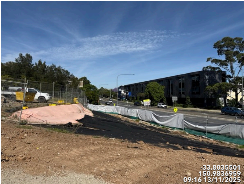
Photo 24 Silt Fence and Geofab were Installed Along the Batter.
