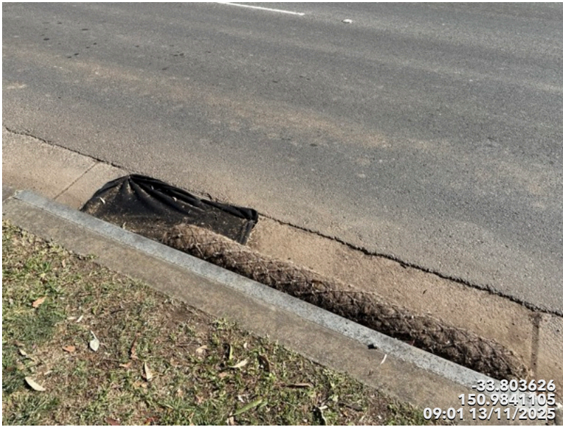
Photo 1. Pits were covered with Geofab and coirlogs were also Installed
