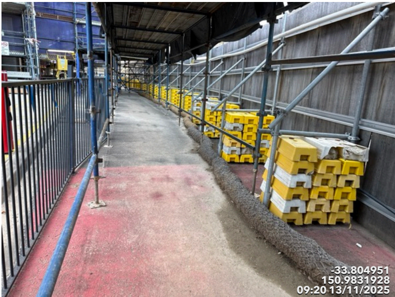
Photo 28 Coir Logs were Installed Around The Perimeter
