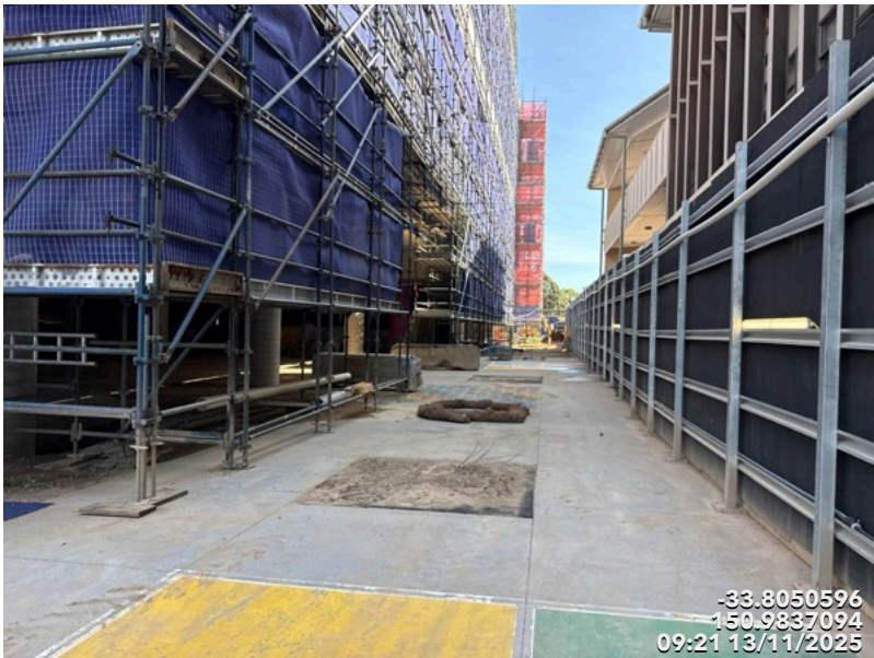
Photo 30 Pits were Covered With Geofab
