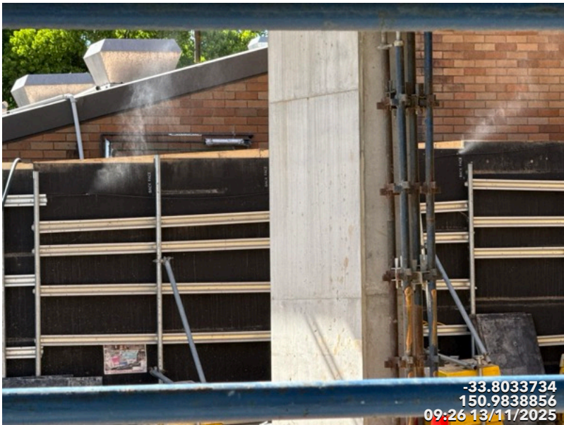
Photo 32 Mist Spray Dust Suppressant
