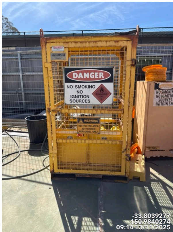
Photo 20 Fuel Storage Is bunded and Labelled
